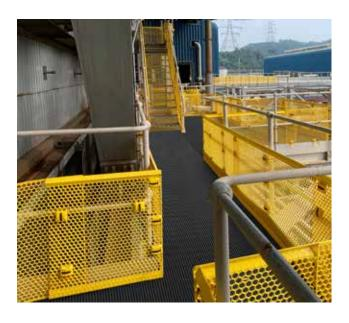
aperture of the barrier panels, prevent loose items falling from height where the barrier is installed.
